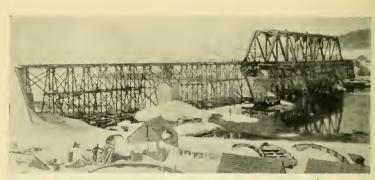
QUEBEC CENTRAL RAILWAY TO THE PORT OF GASPÉ. A long bridge being erected across a wide river. The piers were constructed during the summer; and during the winter the scaffolding was built on the surface of the ice for the erection of the steelwork.
